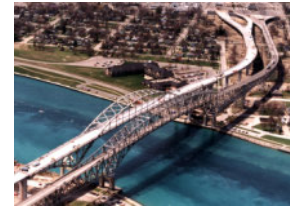
1997 Blue Water Bridge Port Huron, MI
